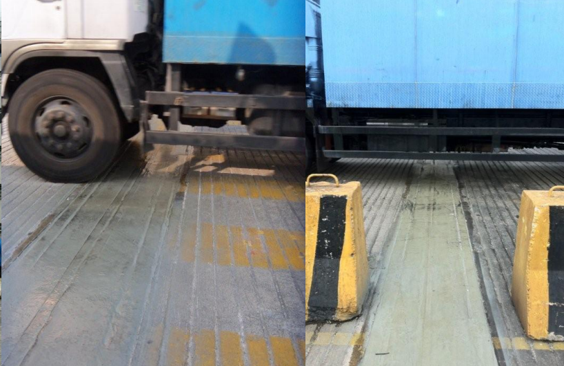
POLYUREA EXPANSION JOINT WATERPROOFING SYSTEM
