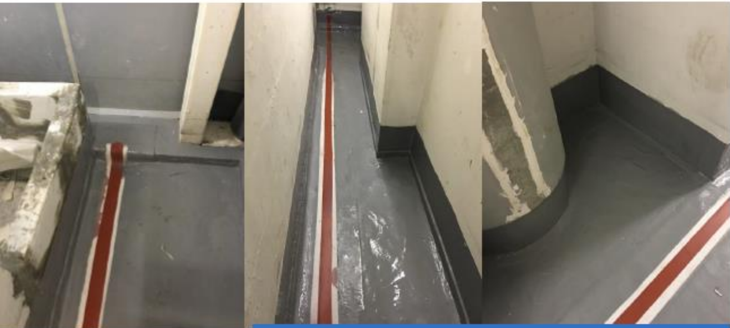
POLYUREA EXPANSION JOINT WATERPROOFING SYSTEM
