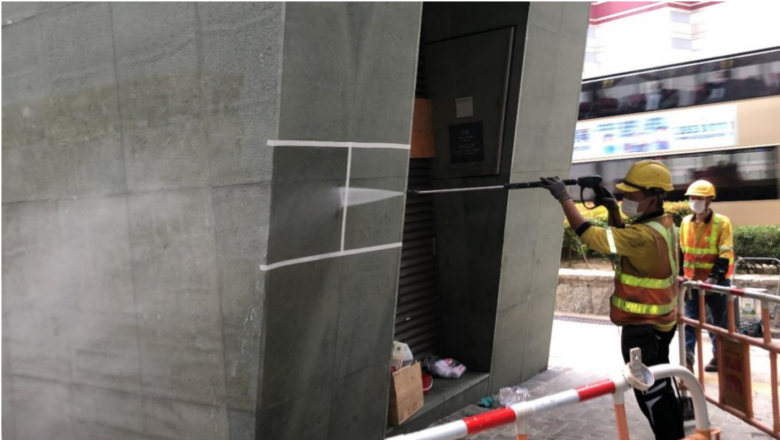
□ Cleaning by Water Jet
