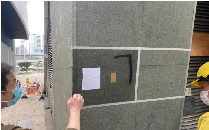
□ Nu-Guard AG surface tested with spray paint / sticker
