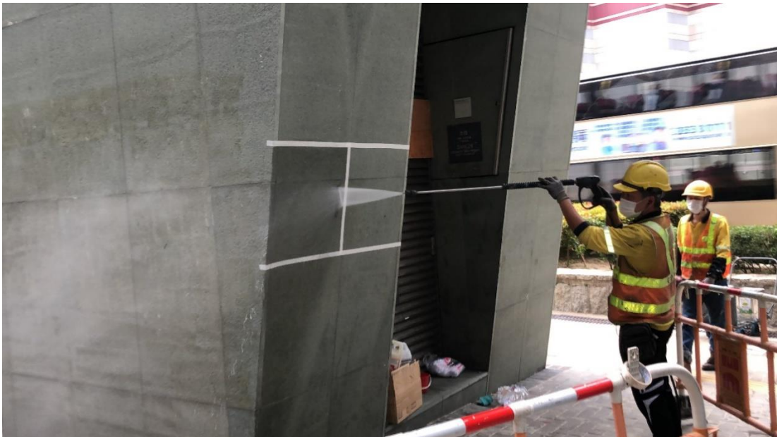
□ Cleaning by Water Jet
