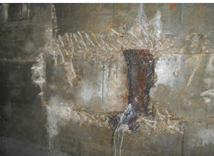
CONCRETE CRACK WAS SEALED UP BY THE CRYSTALLIZATION OF PENETRON AND THE WATER LEAKAGE OF THE CRACK WAS STOPPED AFTER 7- 14 DAYS.
