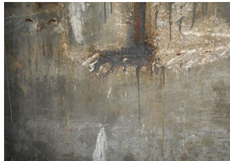
CONCRETE CRACK WAS SEALED UP BY THE CRYSTALLIZATION OF PENETRON AND THE WATER LEAKAGE OF THE CRACK WAS STOPPED AFTER 7- 14 DAYS.
