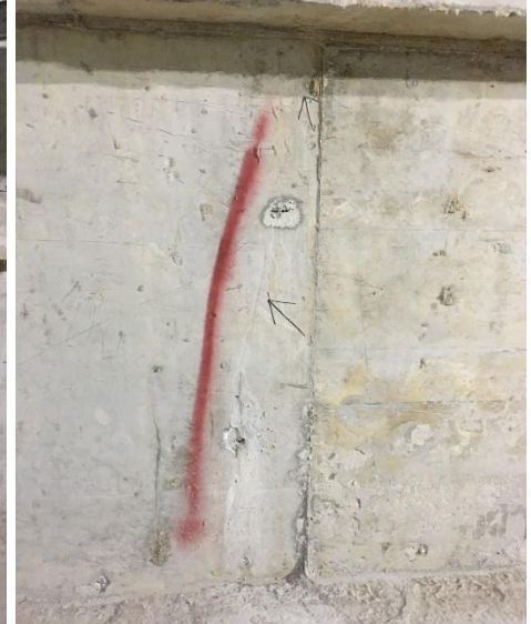
CONCRETE CRACK WAS SEALED UP BY THE CRYSTALLINIZATION OF PENETRON AND THE WATER LEAKAGE OF THE CRACK WAS STOPPED AFTER 14 DAYS.
