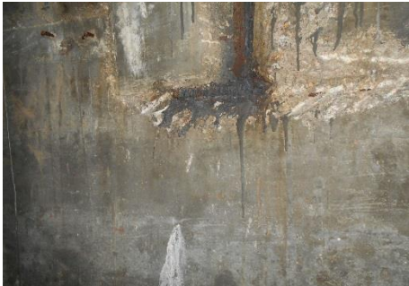
CONCRETE CRACK WAS SEALED UP BY THE CRYSTALLINIZATION OF PENETRON AND THE WATER LEAKAGE OF THE CRACK WAS STOPPED AFTER 7- 14 DAYS.
