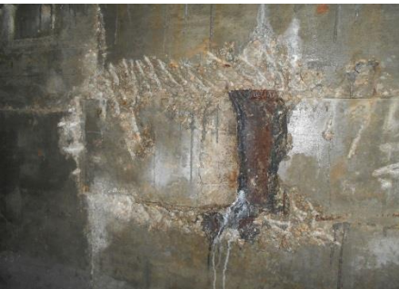
CONCRETE CRACK WAS SEALED UP BY THE CRYSTALLINIZATION OF PENETRON AND THE WATER LEAKAGE OF THE CRACK WAS STOPPED AFTER 7- 14 DAYS.
