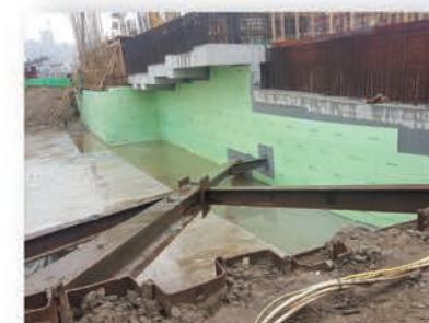
Spray Applied Polyurea Tanking Membrane with Primer for Open Cut
