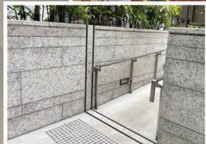
Completed Movement Joints
