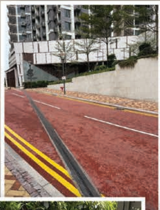
Completed Movement Joints
