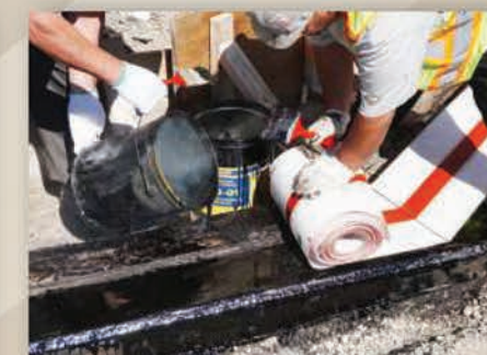
Hot Rubberized Asphalt Installation
