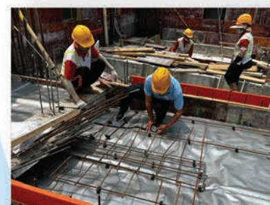
Vapour Proof Membrane for Basement / Ground Slab Underneath
