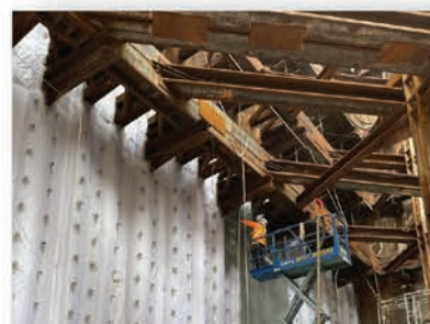
Spray Applied Polyurea Membrane with Geotextile for Blind Side
