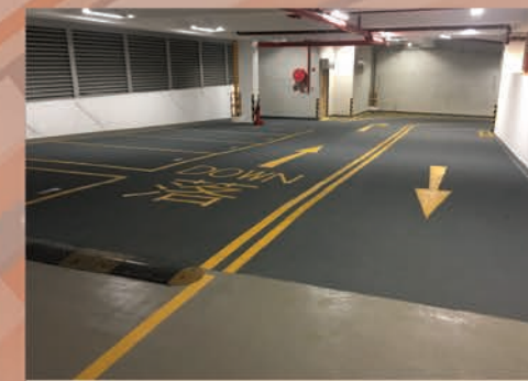
High Skid Resistance Epoxy Resin Flooring System - For Car Ramp
